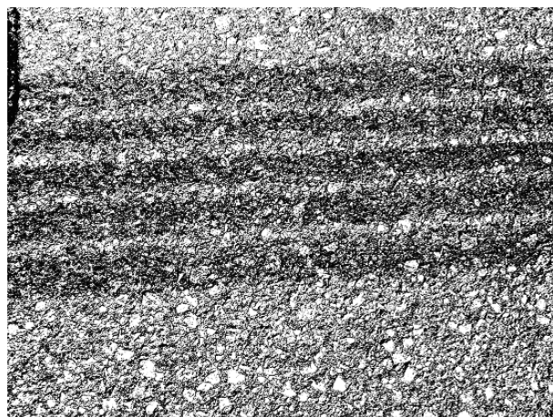
FIG. 1—Short section of skid mark on concrete road with gravel aggregate.
